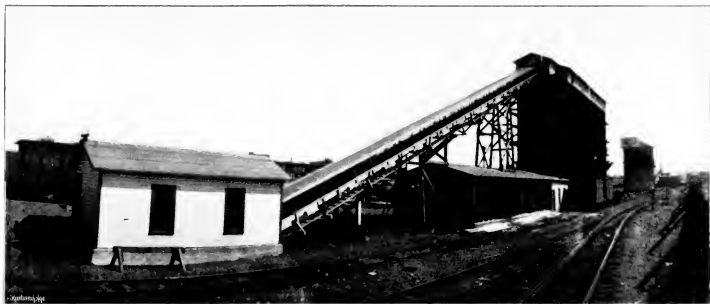
CENTRAL OF NEW JERSEY LOCOMOTIVE COALING PLANT—COAL WHARF AT ELIZABETHPORT, WITH ROBINS BELT CONVEYOR.
